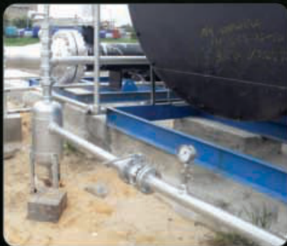
Gas Heater for Gas Supply System
