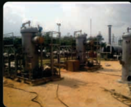
Gas Heater for Gas Supply System
